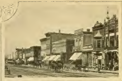
View on East Court St.
